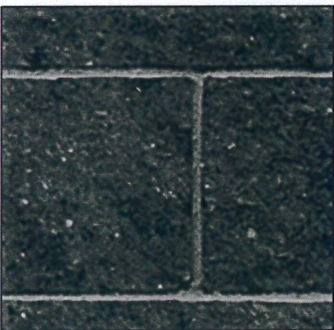
CMU-1 - 8X8X16 INTEGRAL COLOR BLOCK, SPLIT FACE - COLOR OPAL
